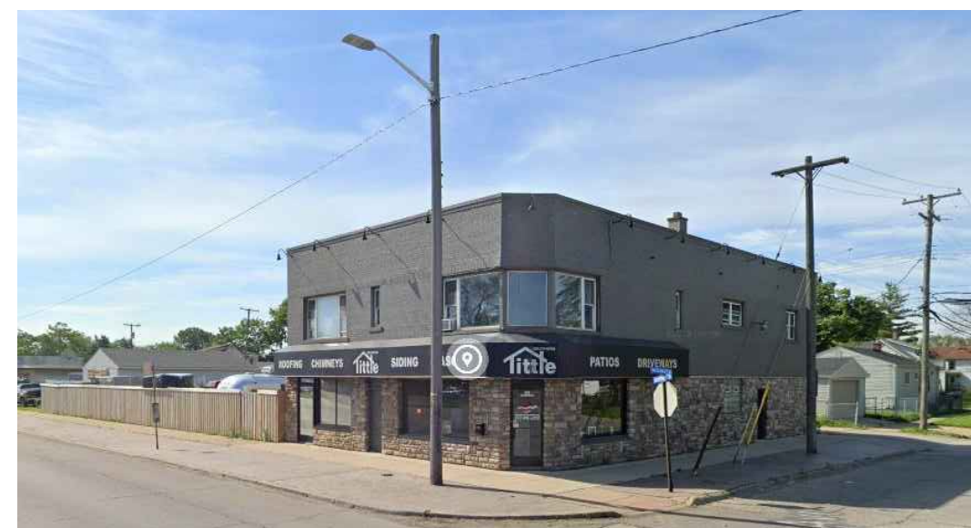
EXISTING BUILDING PHOTO
