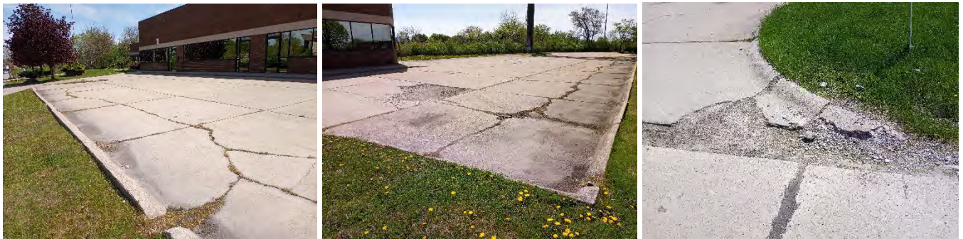
Figure 5: Existing conditions of parking lot and curbs.
