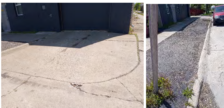
Figure 6: Existing concrete and asphalt conditions.
