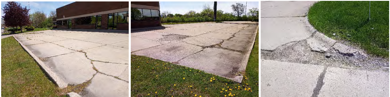
Figure 5: Existing conditions of parking lot and curbs.
