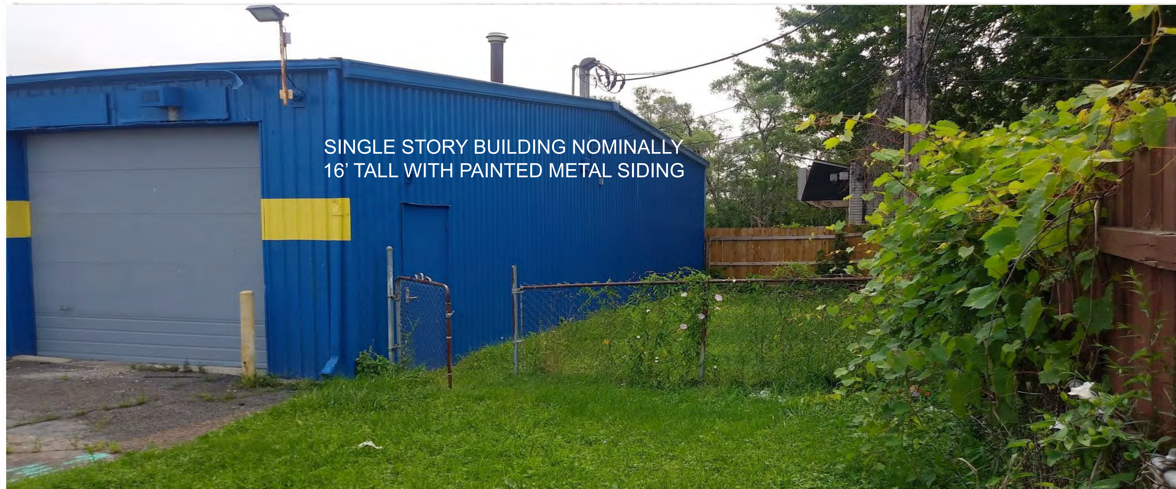
REAR (WEST) ELEVATION showing North-West corner
