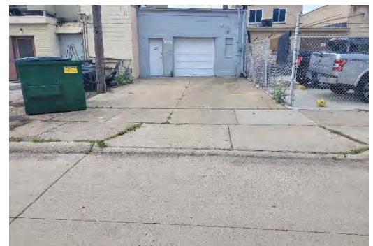
Figure 6: Parking area at back of building.
