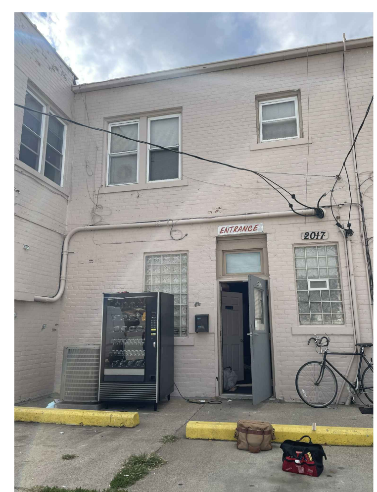
EXISTING REAR ENTRANCE 8
