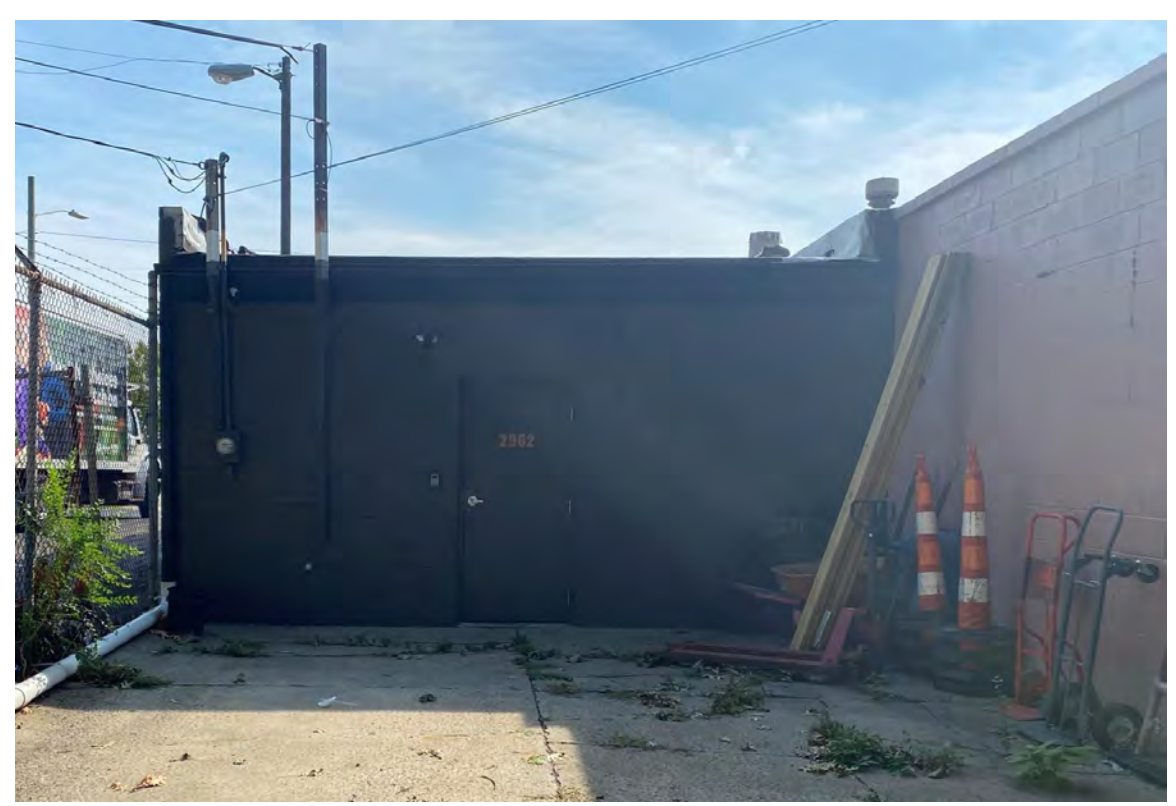
Image of west elevation
