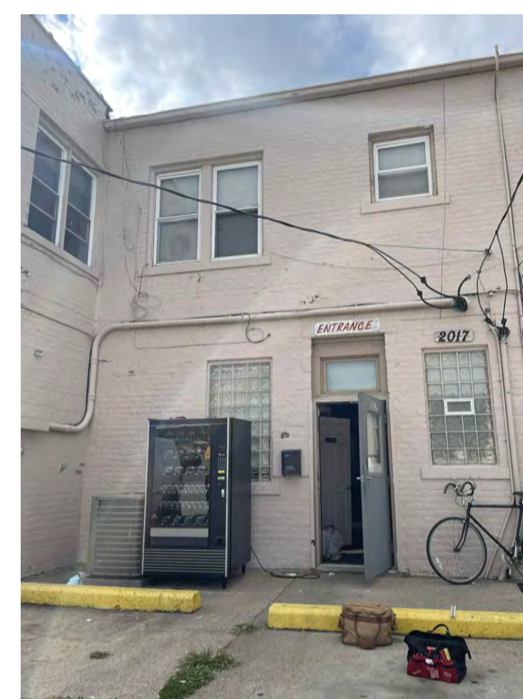
EXISTING REAR ENTRANCE
